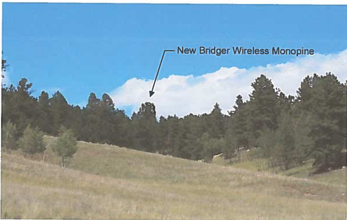
New Bridger Wireless Monopine w/ Future Antennas
